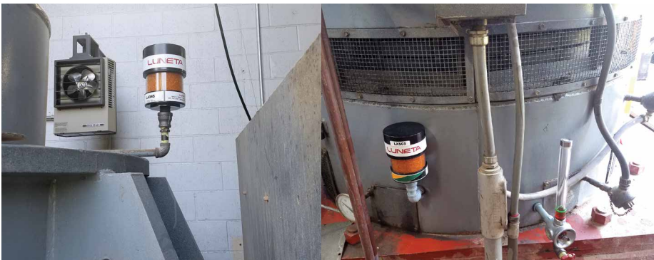
Large Motor - Water Treatment Plant
