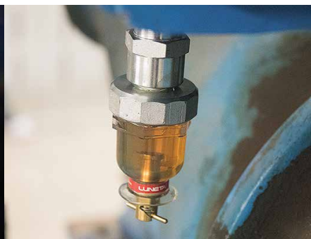
Large Blower - Wastewater Treatment Plant
