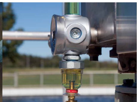
Clarifier - Wastewater Treatment Plant
